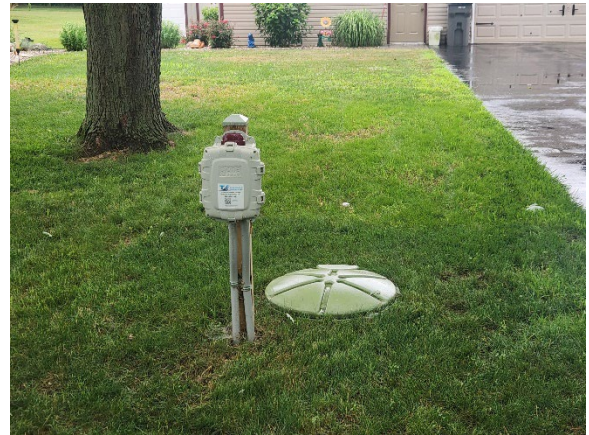
Grinder Station and Alarm Box
